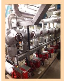
New low temperature hot water pumps with inverters and bespoke insulation jackets have been installed as part of the £1.1 million energy saving upgrade
