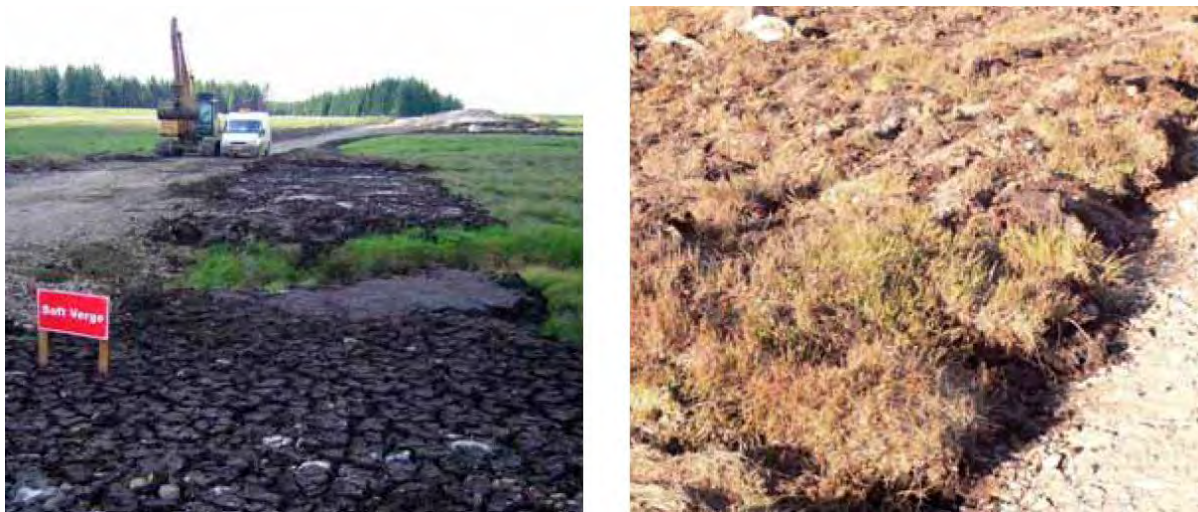
Photograph 2 Poor (left) and good (right) reinstatement of track verges (Scottish Renewables et al. 2015)
