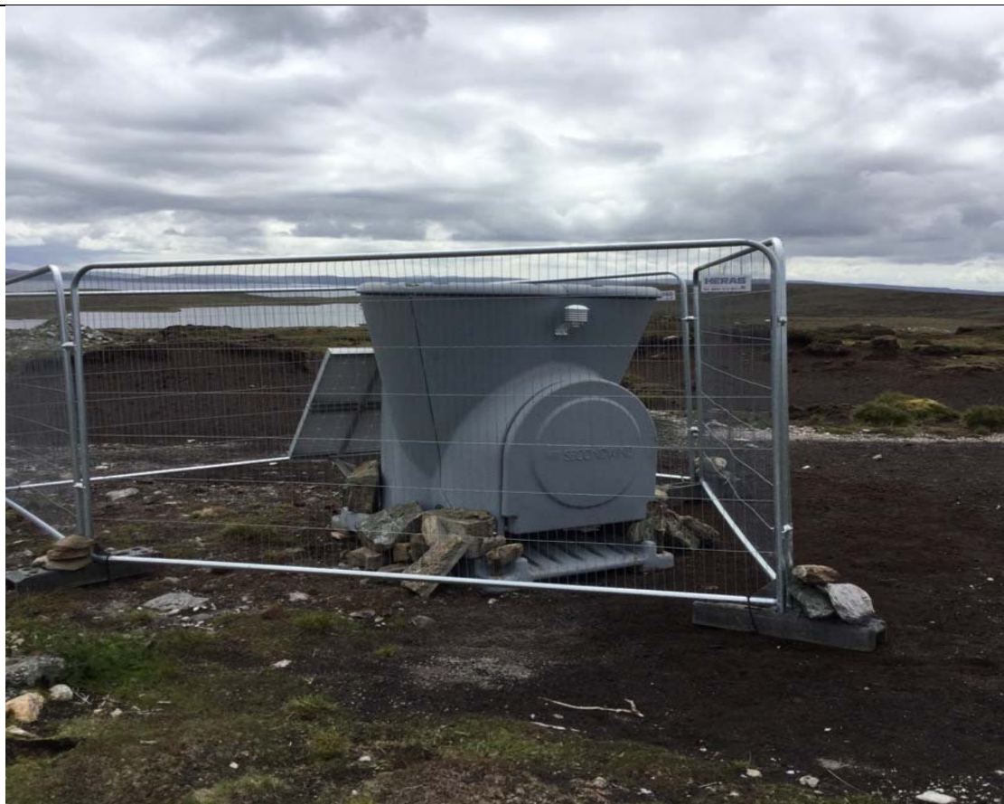
View towards Triton, looking South-west
