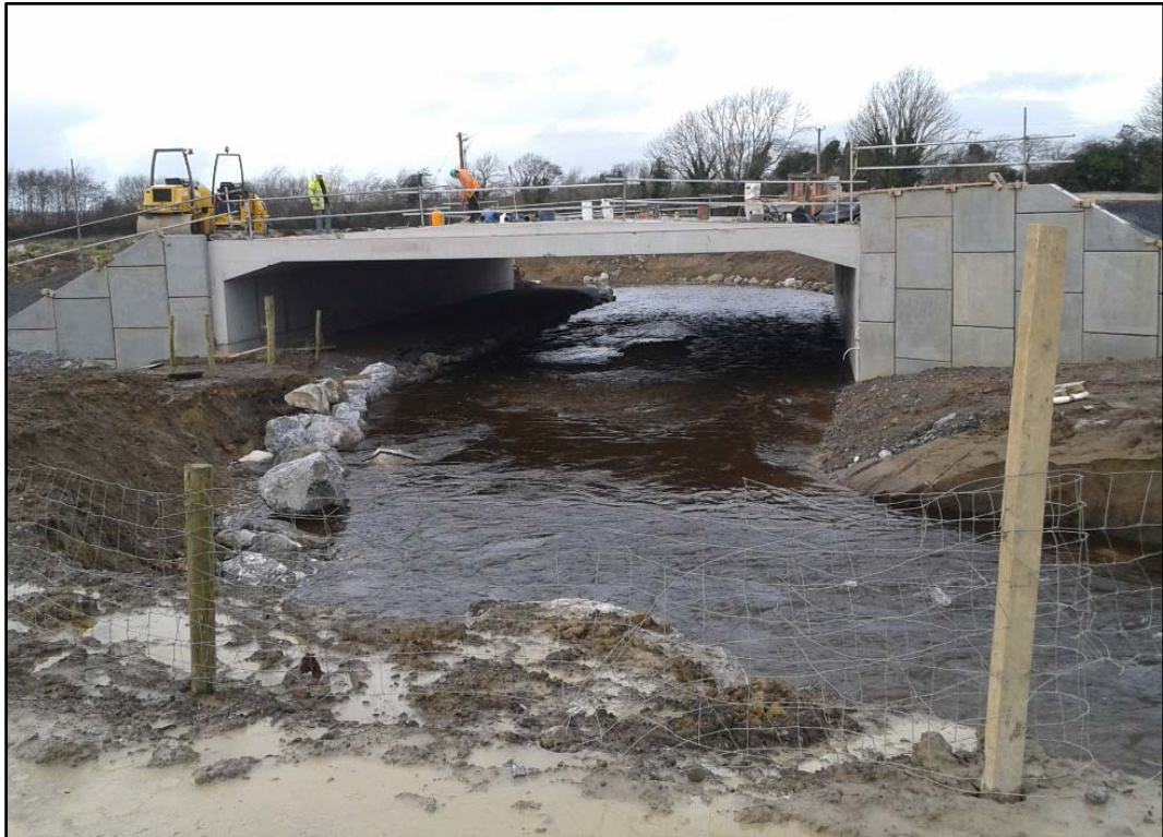
Plate 3: Example of a large span portal frame bridge (Image courtesy of Banagher Precast)
