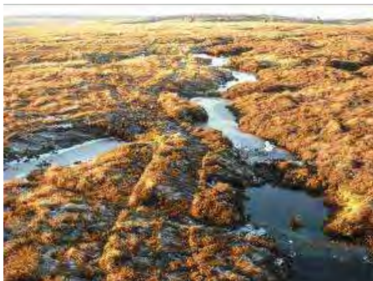
Photograph 4 Series of bunds and dams in a gully (from gully blocking undertaken in East Ayrshire, 2008)
